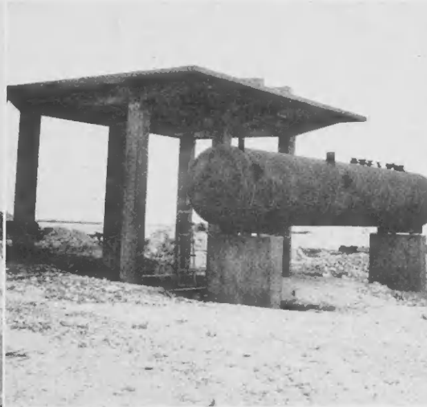
A GOVERNMENT substation will take high voltage electricity from the government system and transform it down to 4160 volts before directing it to the Antilles switch house, above left. Transformers of the ammonia company will adjust the power to fill Antilles' varied electric needs. The group of structures above will support the urea plant condensers of ACI.
